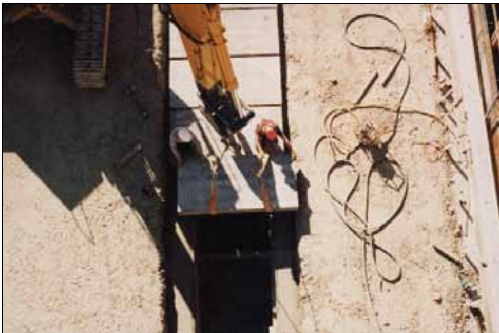
Figure 5 - Placing Precast pre-tensioned panels
