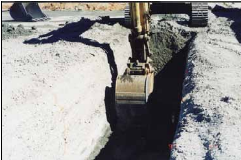
Figure 1 - Excavation of Gallery
