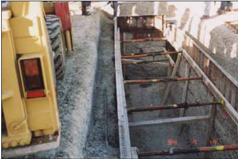
Figure 2 - Forming of edge beams
