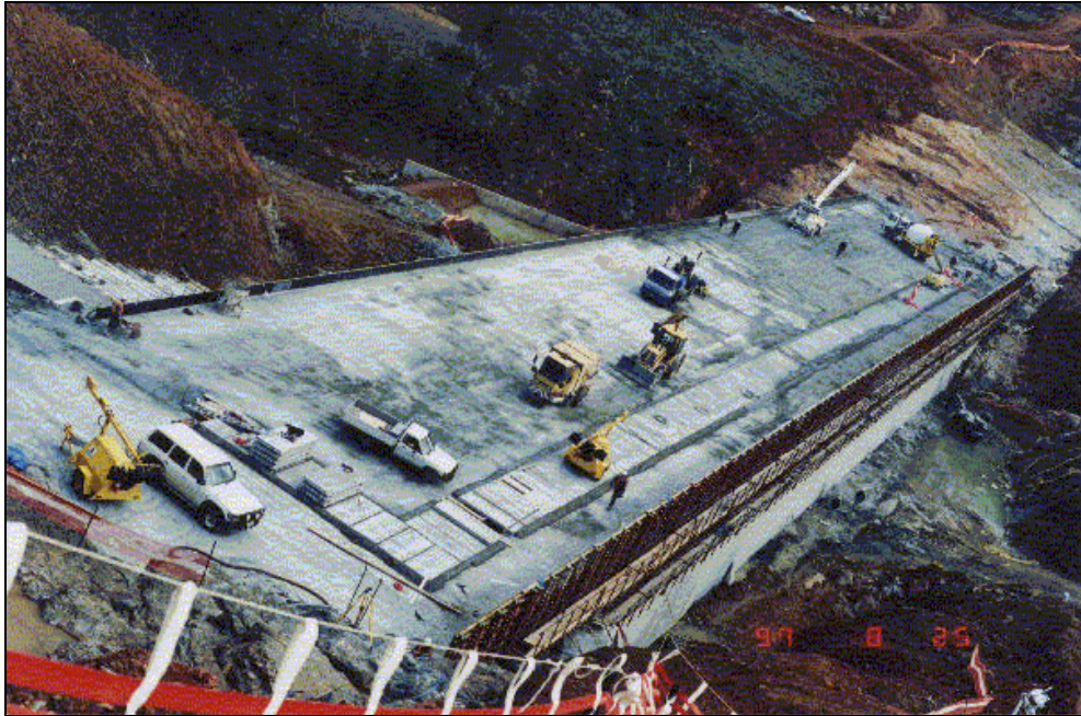
Figure 6 - Top surface of gallery following installation of precast panels
