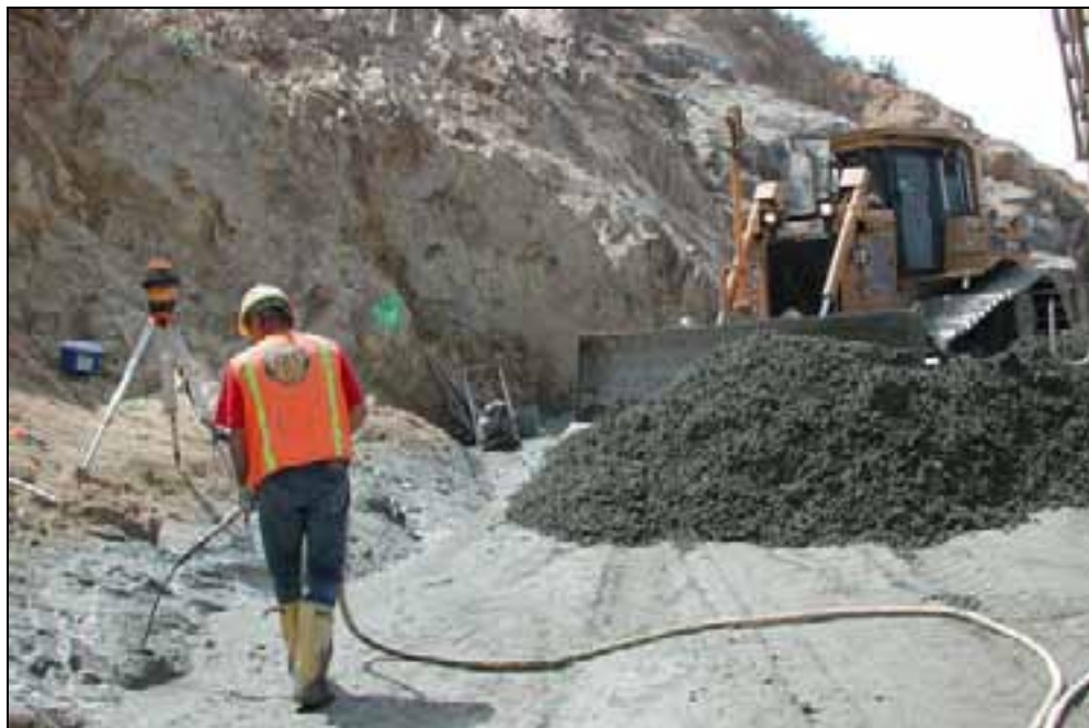
Spreading grout against an abutment at Olivenhain dam
