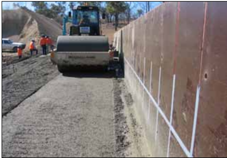
Rolling the interface between parent RCC and the grout enriched zone
