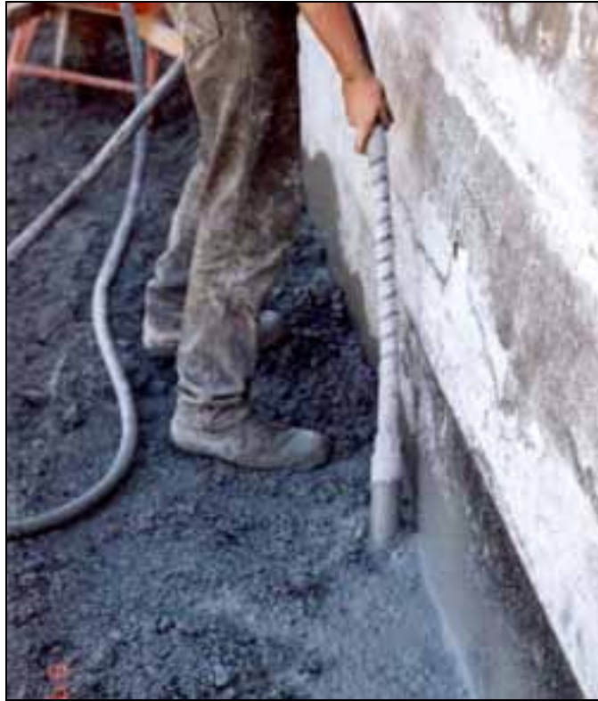
Typical View of Immersion Vibration of Grout Enriched RCC
